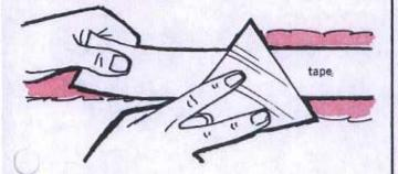
Next, take your wallboard tape, center it over the joint and press the tape firmly, into the bedding compound with your wall-board knife held at a 45° angle. The pressure should squeeze some compound from under the tape, but enough must be left for a good bond.
